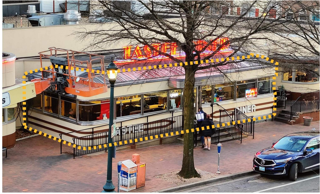
EXISTING AERIAL VIEW
