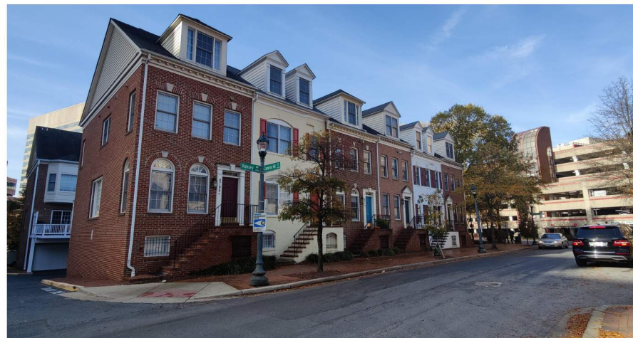
3 VIEW FROM RAMSEY AVE LOOKING NORTHWEST
