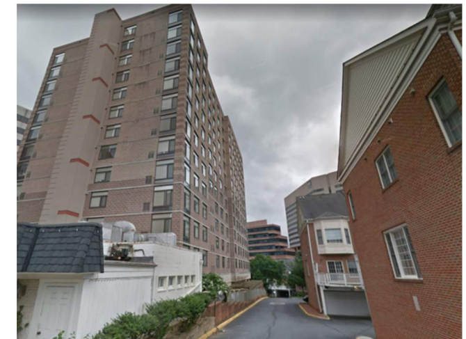
8 RAMSEY AVENUE LOOKING WEST
