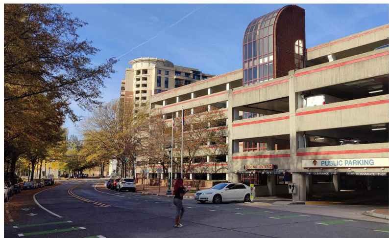
6 VIEW FROM CAMERON STREET LOOKING WEST
