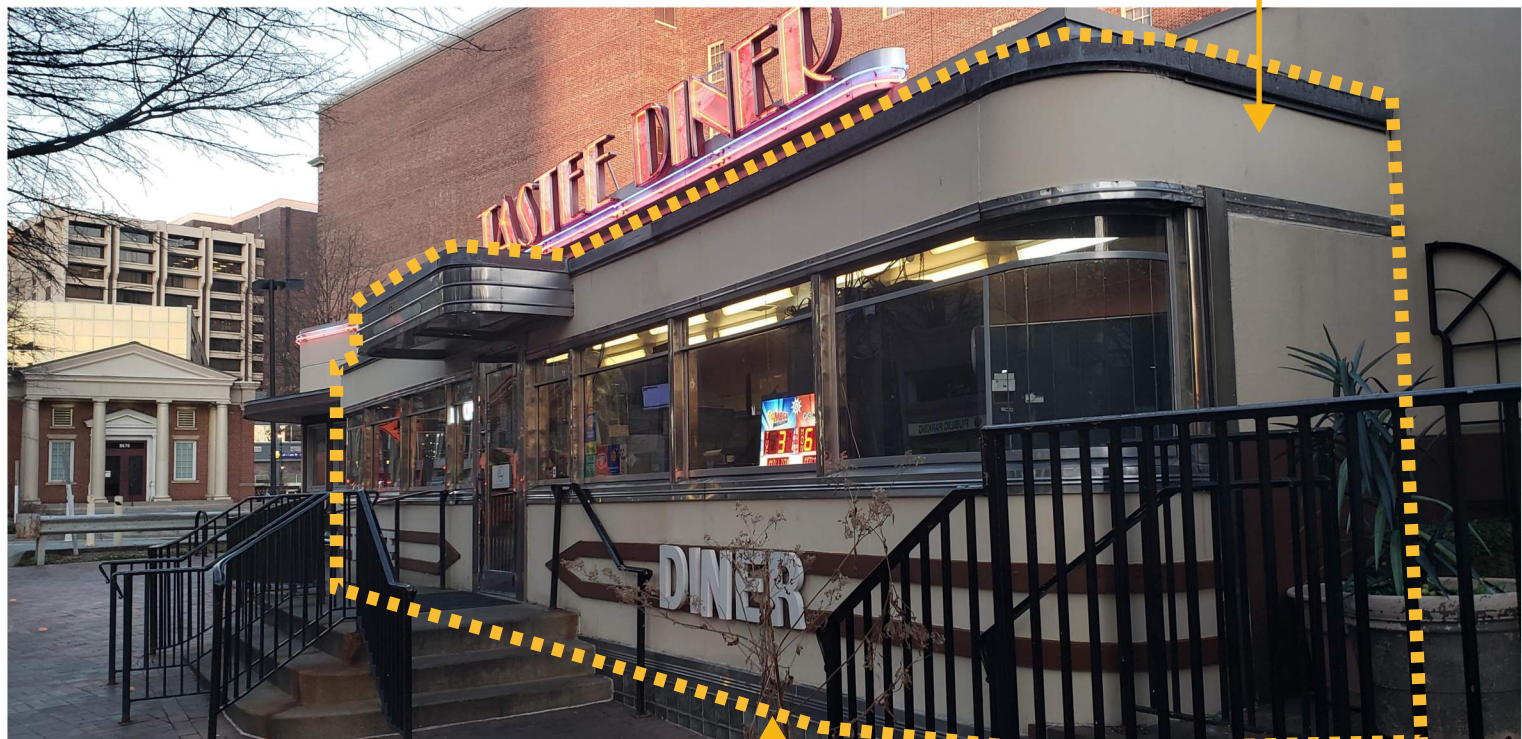
EXISTING VIEW FROM NORTHWEST
